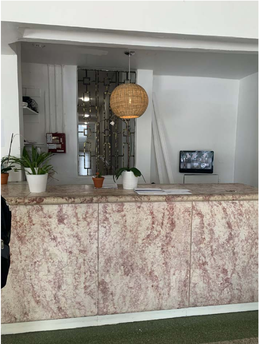
1 LOBBY EXISTING CONDITIONS
