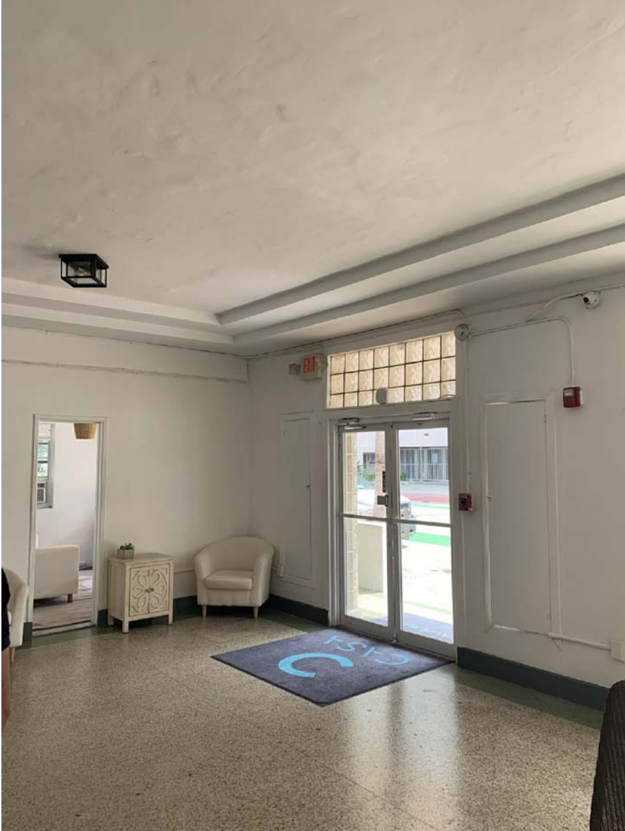
3 LOBBY EXISTING CONDITIONS
