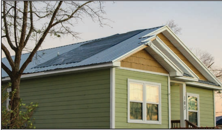
Figure 8: Successful sealed roof deck (Panama City area)
