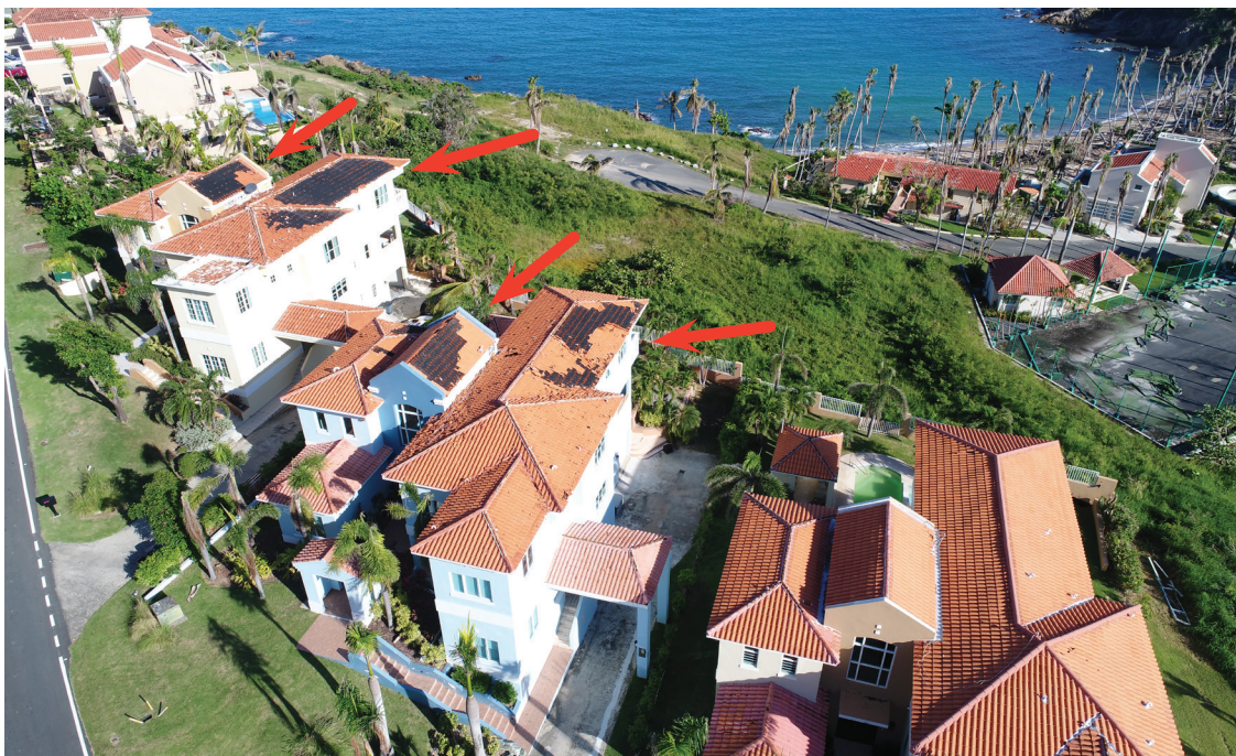
Figure 3-2: Roof damage from wind speed-up effects
