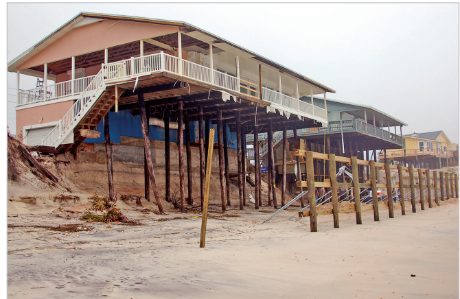
Figure 3-1: Undermined houses constructed on top of the dune in Vilano Beach, FL.
