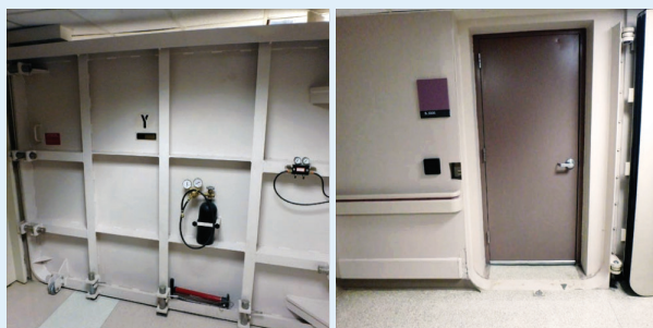
Flood doors in basement that subdivide basement areas within the main building.
