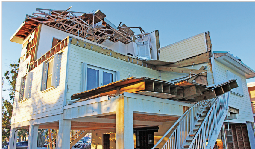
Figure 3-8: House with wind damage.
