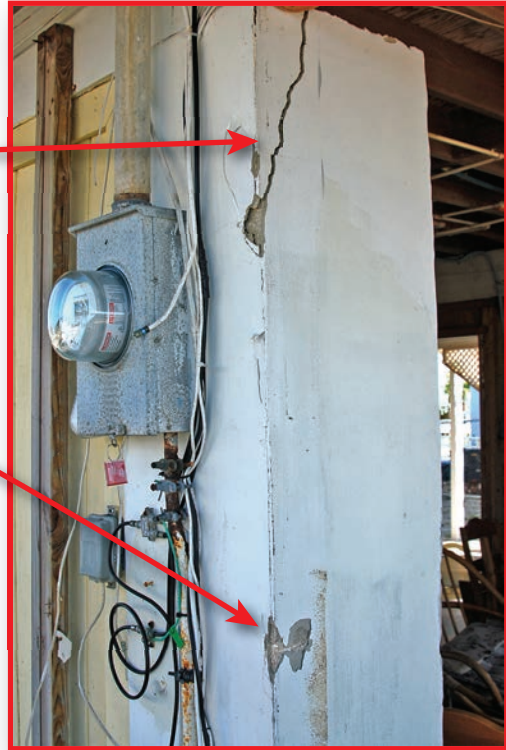
Figure 3-9: Example of a breakaway wall failure that likely contributed to damage to columns (Big Pine Key, FL)
