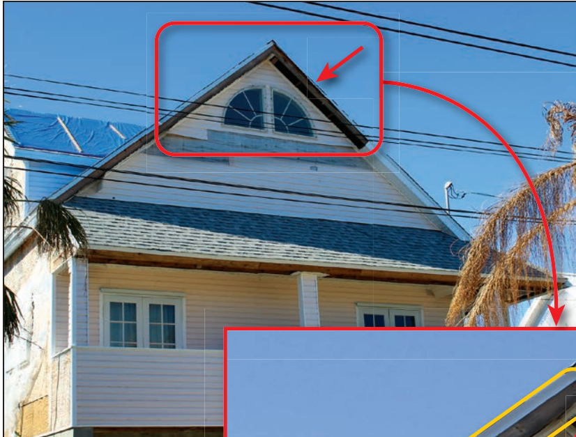
Figure 4-18: House that lost its soffit along the right side of the front-facing gable (EWS = 114 mph; EDWS = 180 mph) (Little Torch Key)
