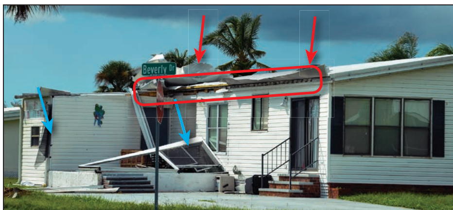
The screened porch (remnants shown with blue arrows) opened the top of an exterior wall (red outline) and peeled back the adjacent roof section (red arrows) when the porch was lost to high winds.
