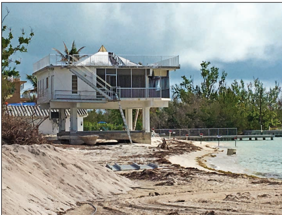
Figure 3-16: Erosion was likely due to wave attack around the foundation of this house on Sombrero Beach Road (Marathon, FL)
