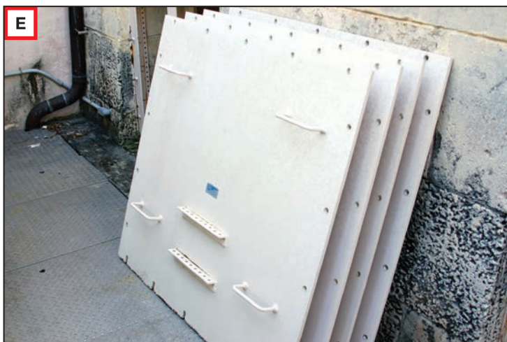
Figure 3-32: Floodproofing system components at a historic building (top); parts of the system failed and approximately 3 feet of flooding infiltrated part of the building (Miami, FL)
