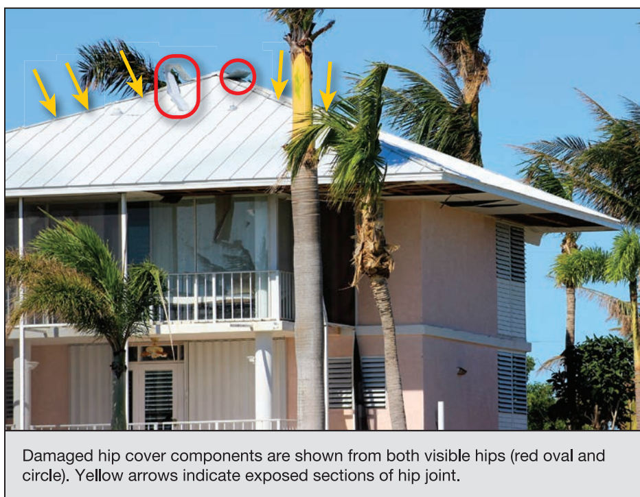
Figure 4-16: House with damaged metal roof system (EWS = 113 mph; EDWS = 180 mph) (Sugarloaf Key)
