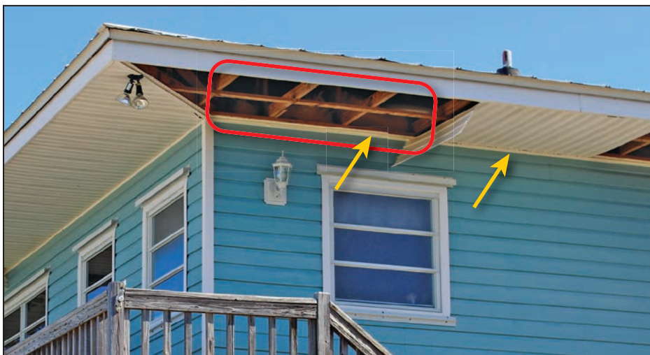
Figure 4-19: House with vinyl soffit damage not caused by fascia loss (EWS = 113 mph; EDWS = 180 mph) (Sugarloaf Key)
