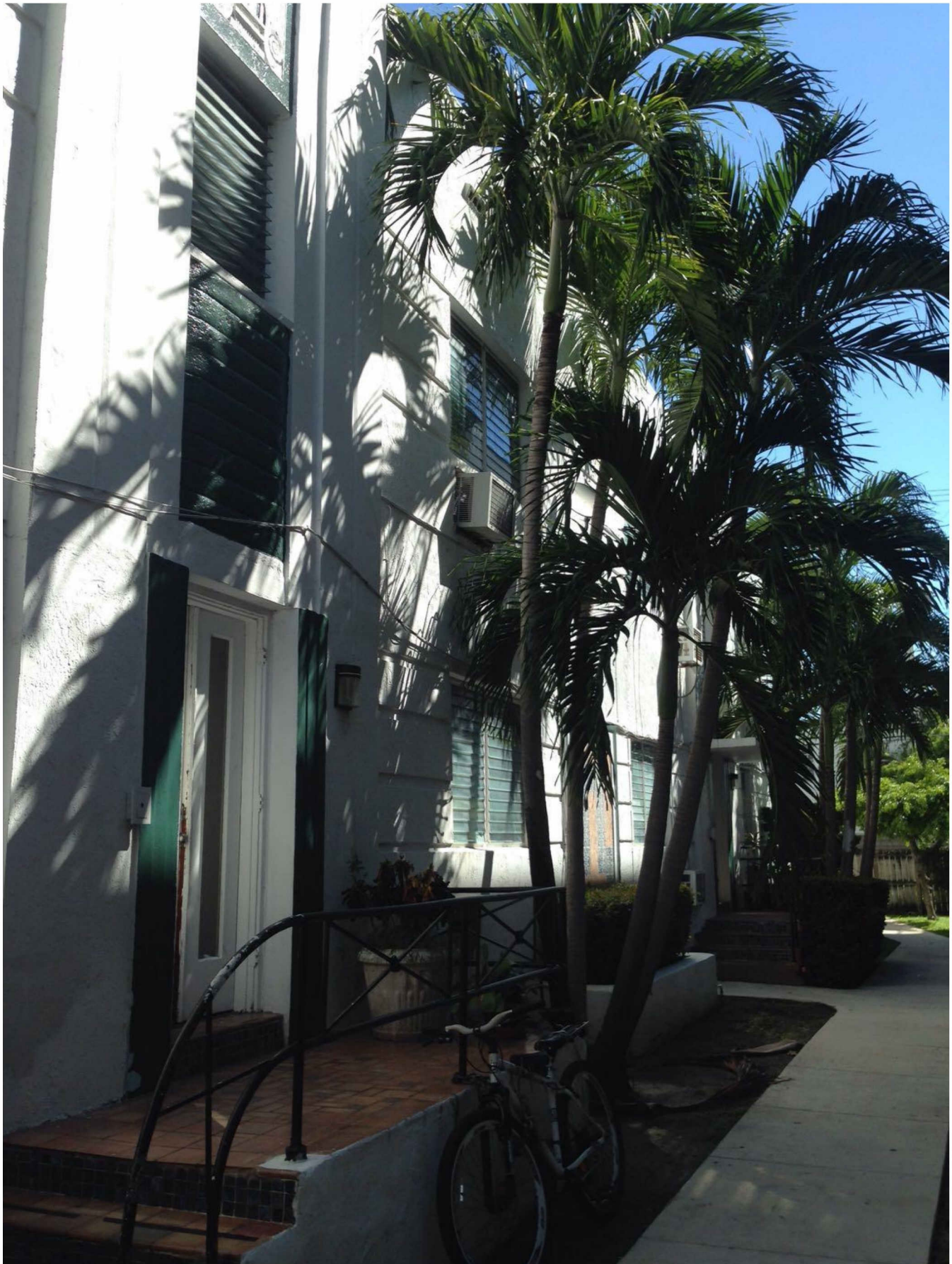
Right side view (3 entrances to the building)
