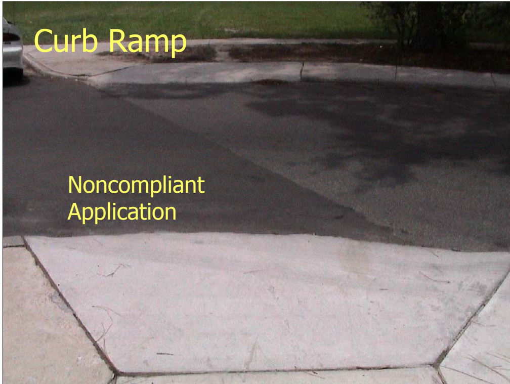
Curb ramp with no detectable warnings of any sort.
