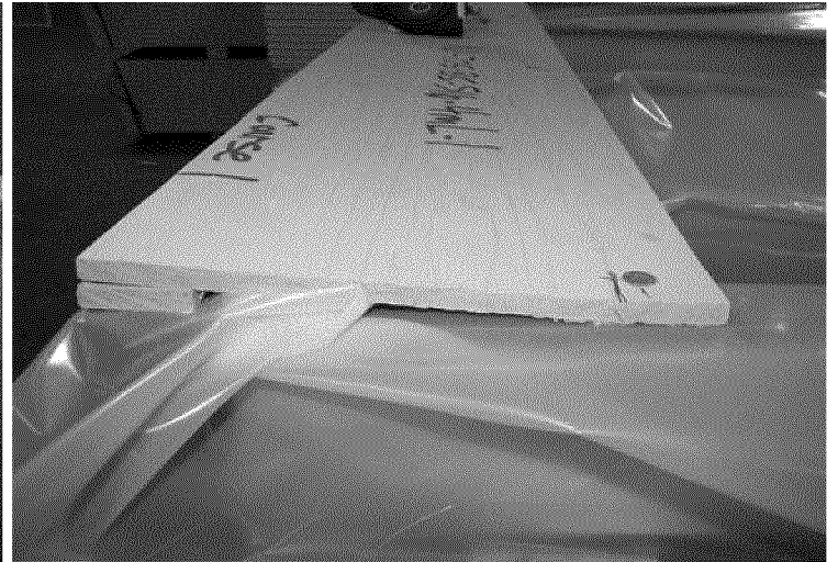
Corner Fastener Installation - Typical
