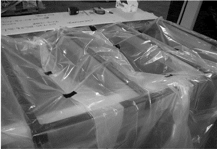
Typical folds in each stud bay - Loose Film
