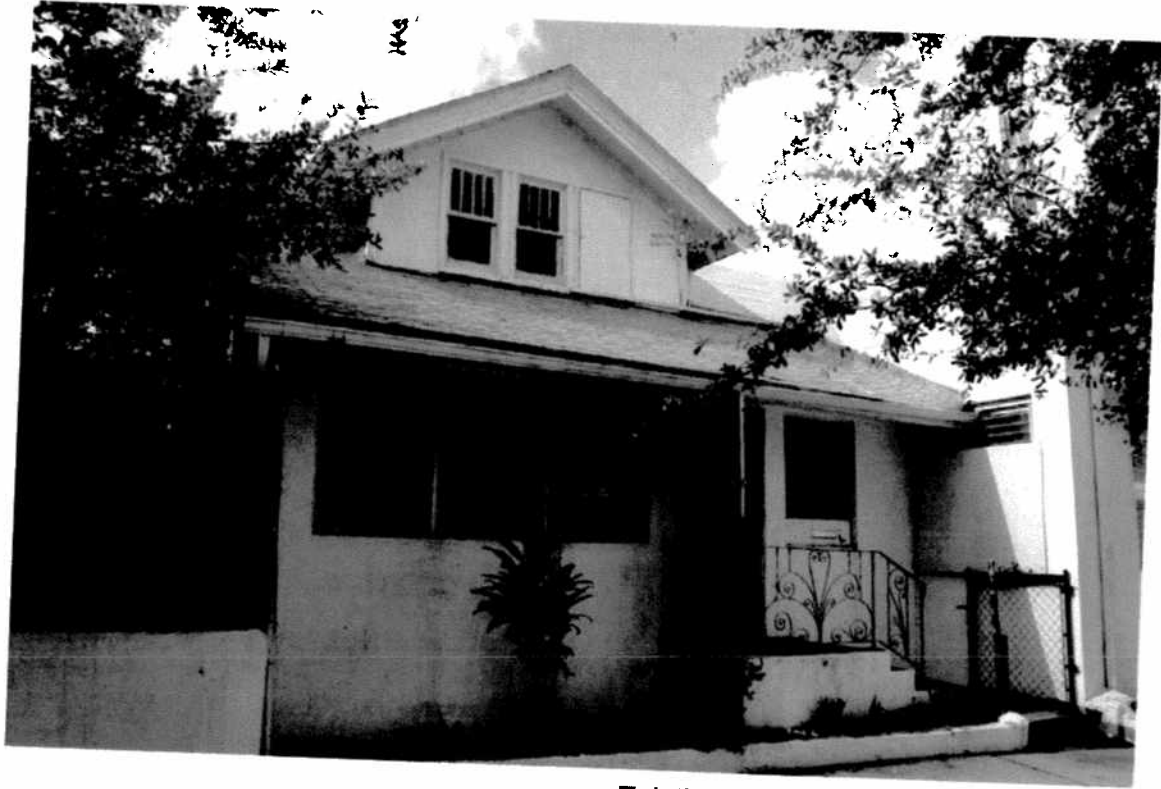
Existing Front Elevation of Bungalow Photo 1
