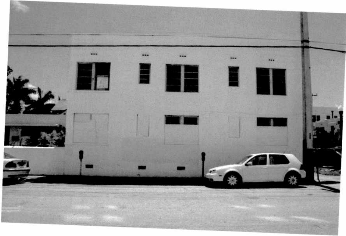
Façade on 4 th Street Photo 5
