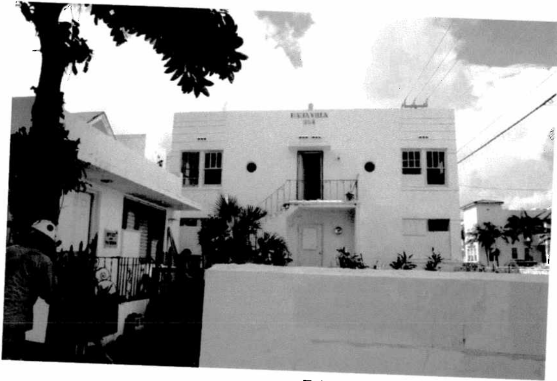
Existing Elevation of 2 Story Hotel Photo 3
