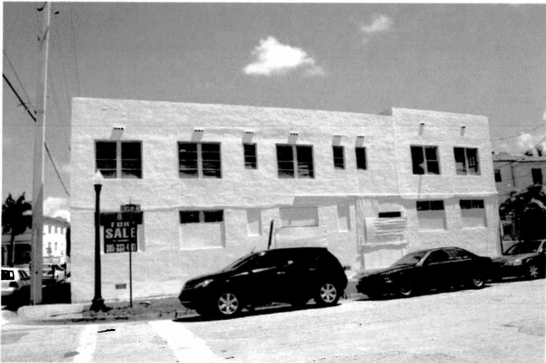
Rear Façade on Euclid Ave Photo 6
