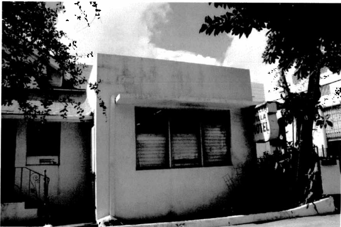
Existing TV Room on Front Elevation Photo 2
