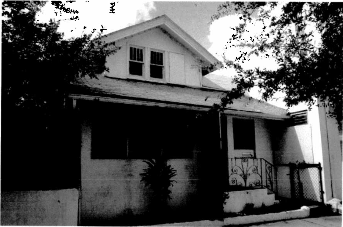
Existing Front Elevation of Bungalow Photo 1
