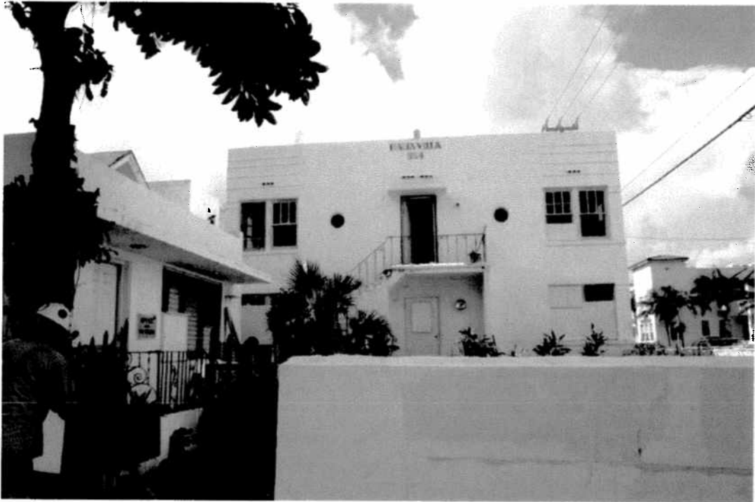
Existing Elevation of 2 Story Hotel Photo 3
