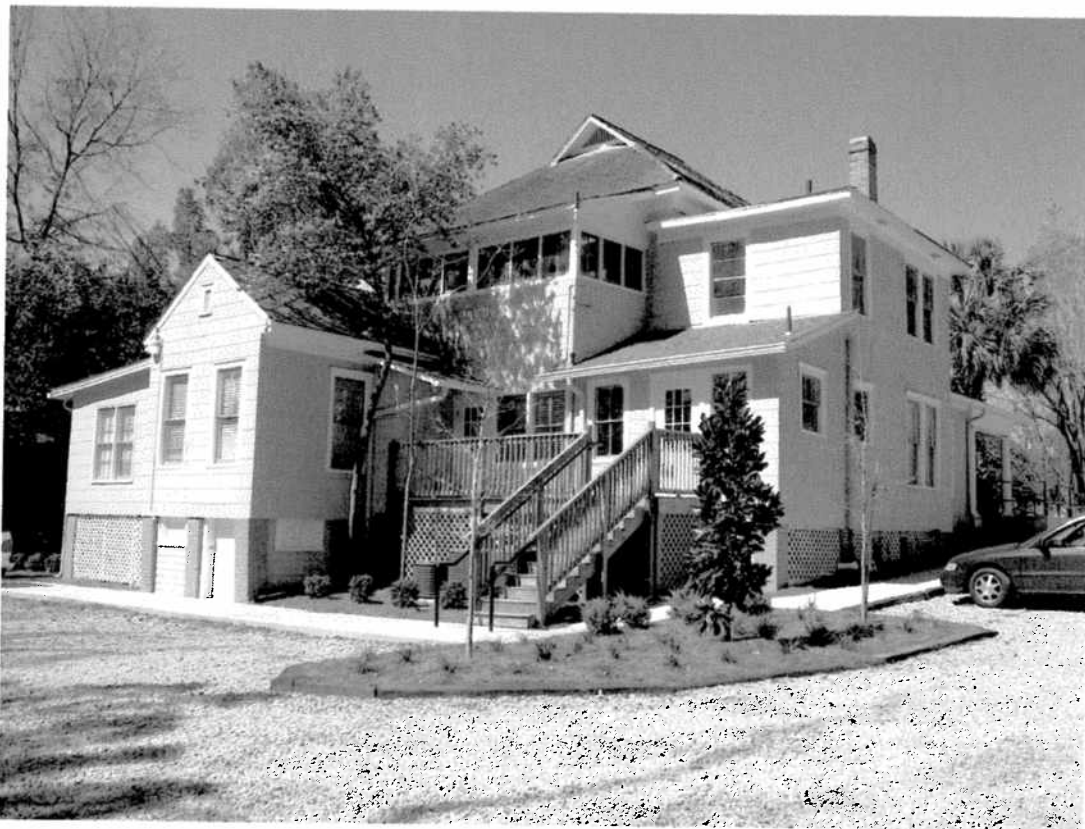
725 East Park Avenue after first floor renovation After new code compliant stairs
