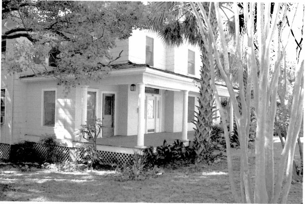
725 East Park Avenue before first floor renovation Before ramp and handicap accessible parking
