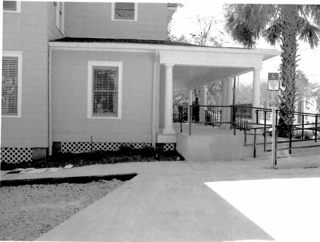
725 East Park Avenue after first floor renovation After new handicap accessible parking
