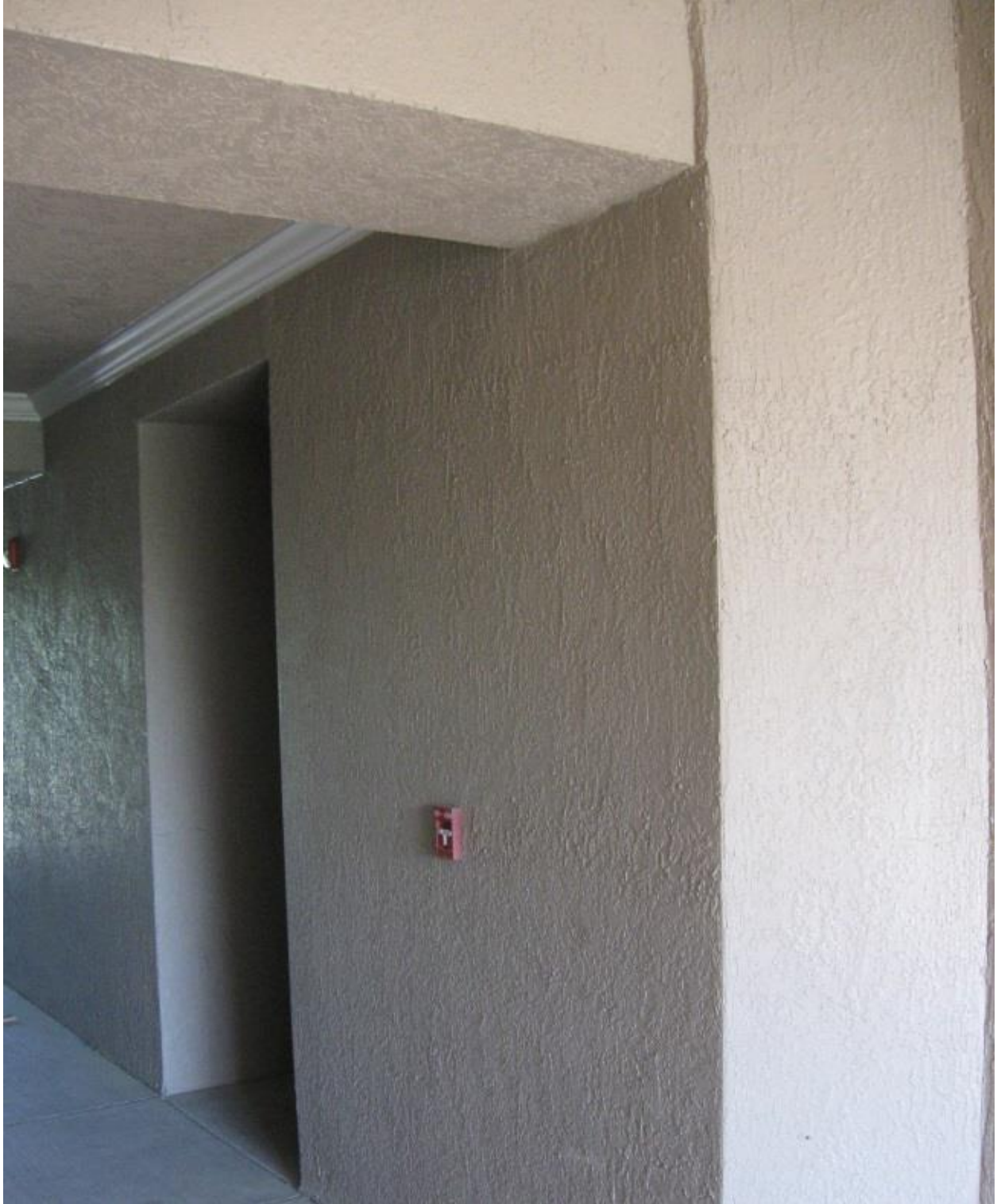
Picture 12 – Building 12 Ceiling Soffit from Breezeway
