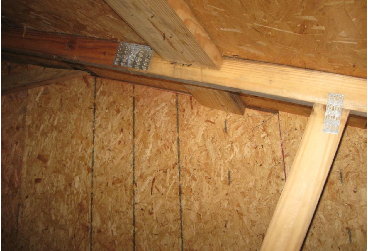
Picture 01 – Typical Plywood Draftstopping
