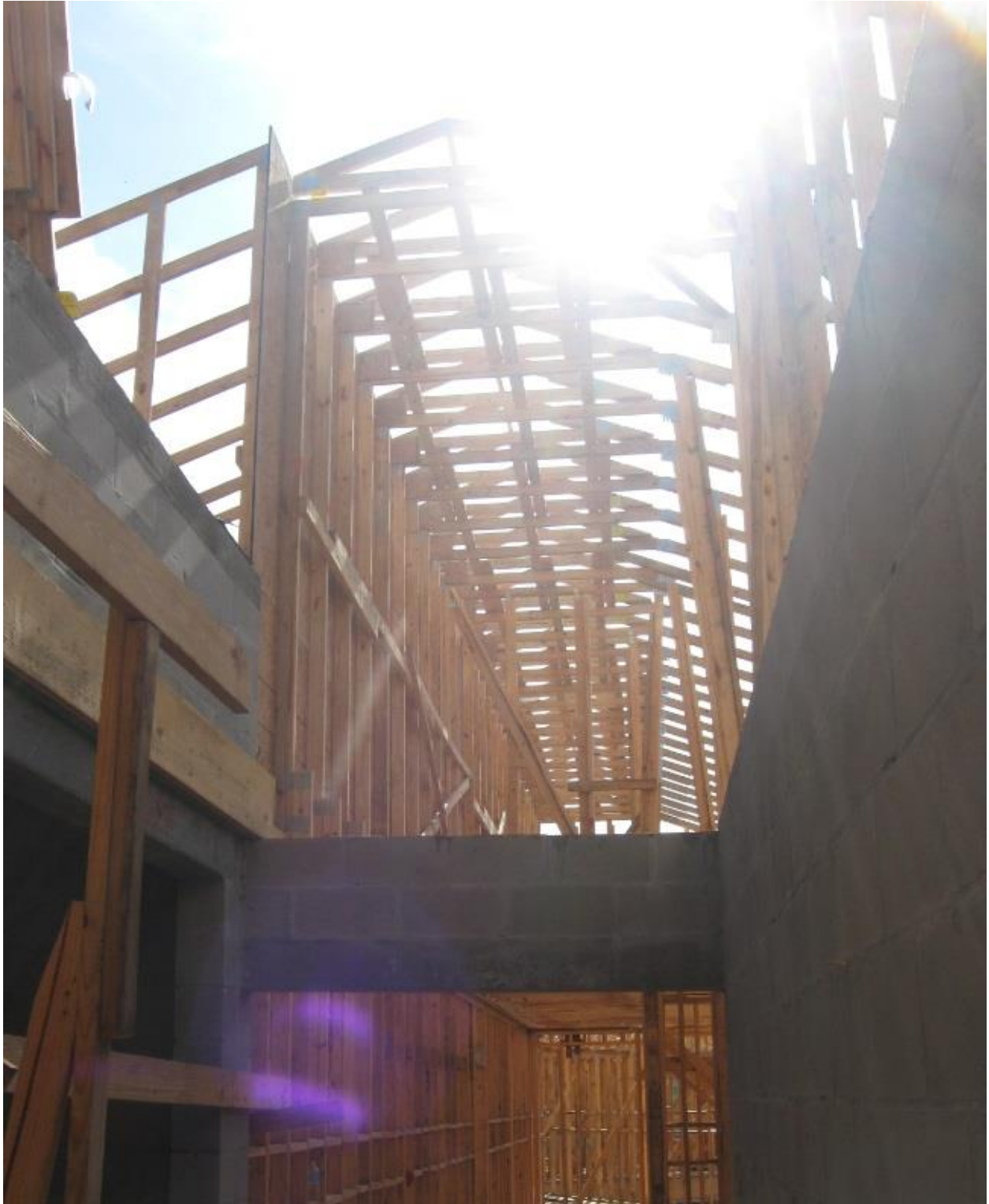
Picture 06 – Draftstopping Installed Perpendicular to the Trusses
