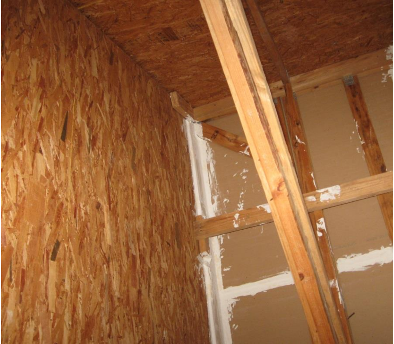
Picture 04 – Draftstopping with both Plywood and Gypsum
