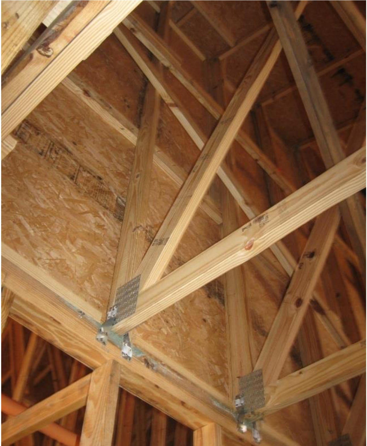
Picture 07 – Draftstopping Installed Perpendicular to the Trusses
