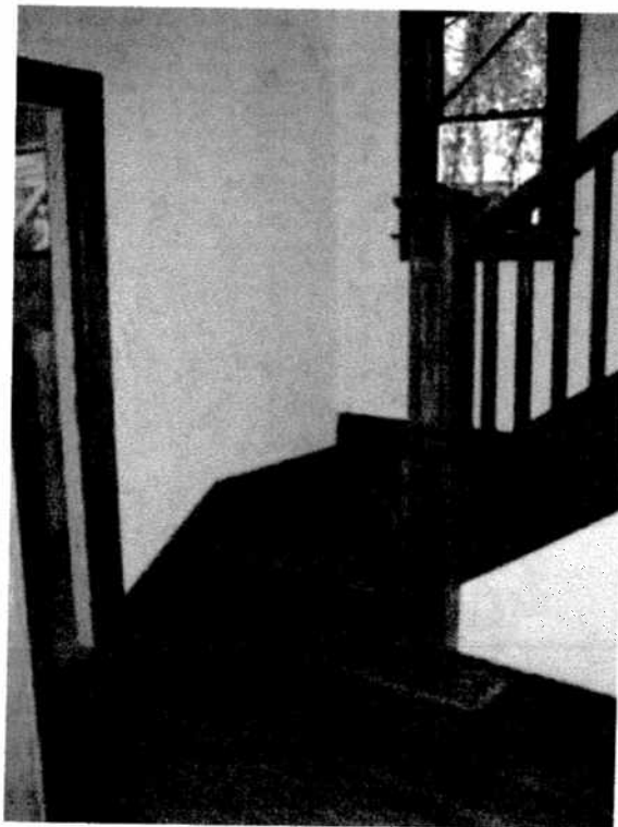
Level One Bottom of Stair
