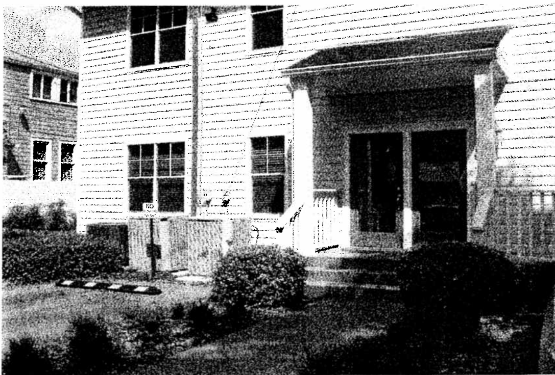
Parking Lot from NW Corner looking at Back Entry & AC Condensers
