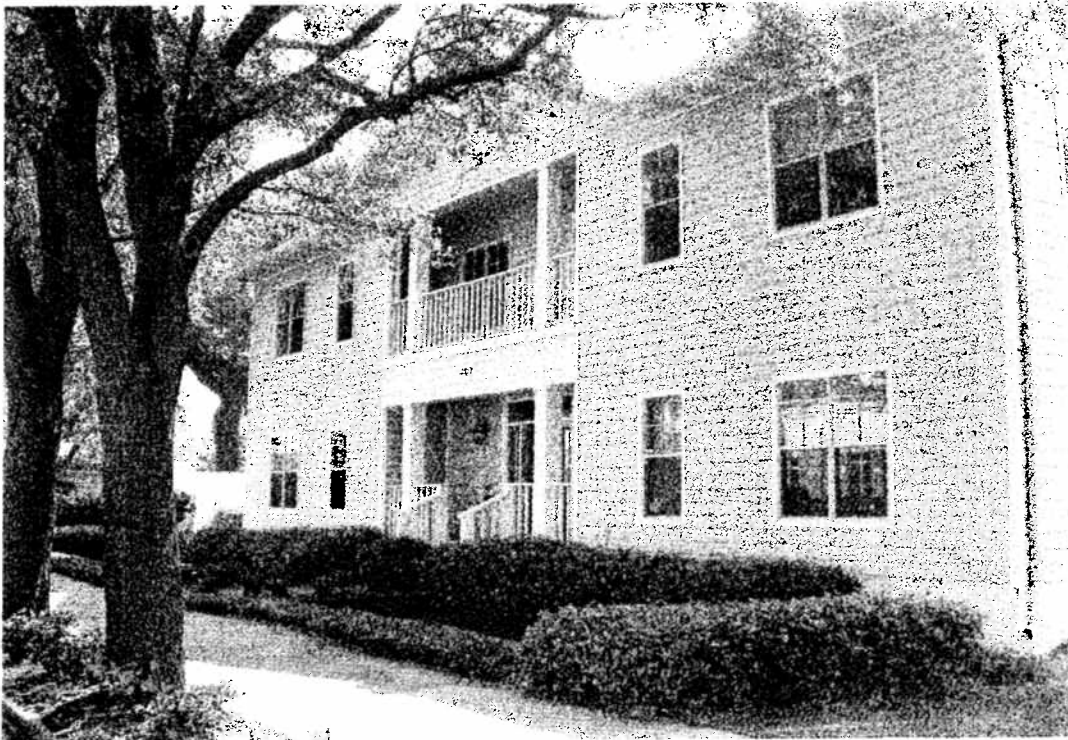
FRONT ELEVATION LOOKING SOUTHWEST
