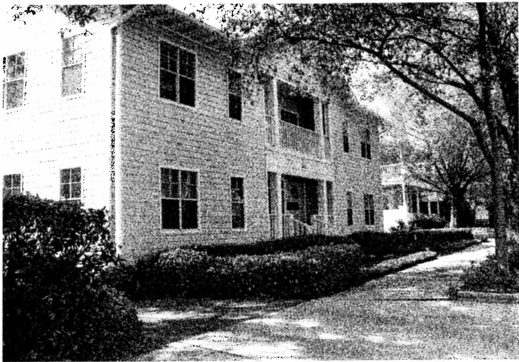
FRONT ELEVATION LOOKING NORTHWEST
