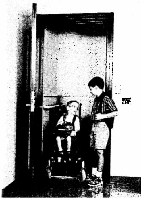
Elementary School: A lift in a fully enclosed hoistway provides lower level access for a kindergartner.
