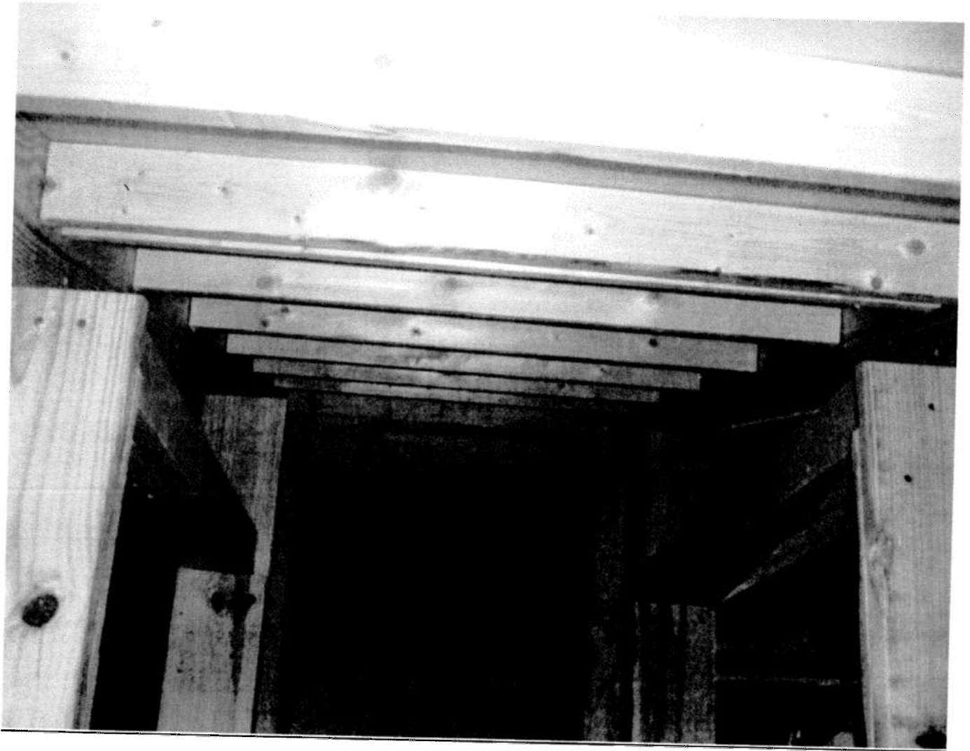
Under Structure of Existing Ramps
