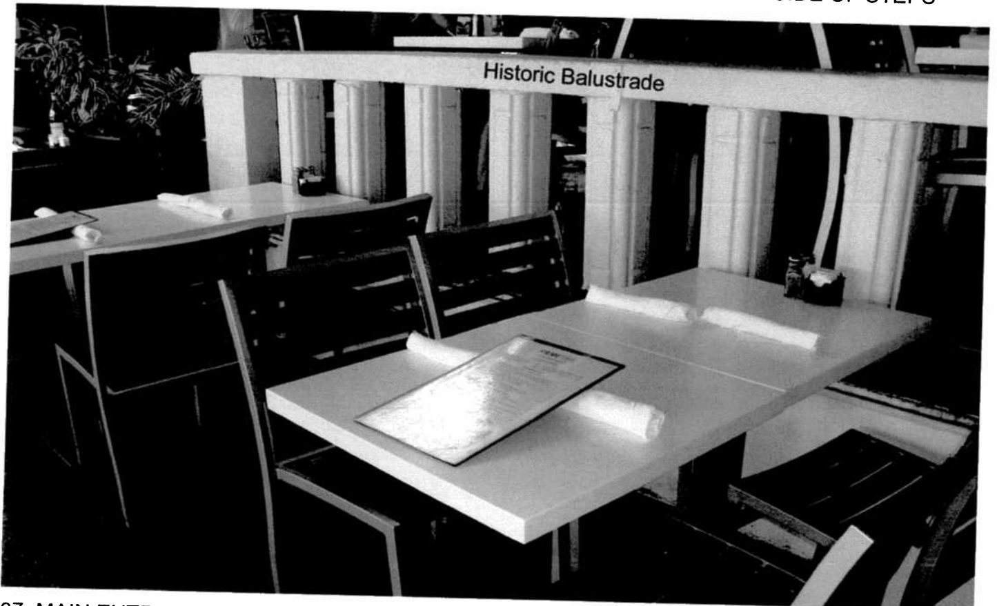
07 MAIN ENTRANCE ON EAST SIDE - VIEW OF HISTORIC BALUSTRADE
