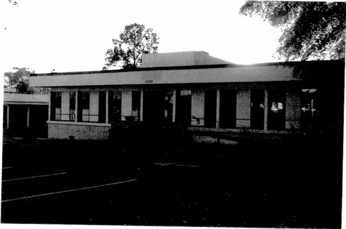
Front of Building
